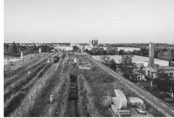
Vegetative roof: an assembly of interacting components designed to waterproof a building's top surface that includes, by design, vegetation and related landscape elements
